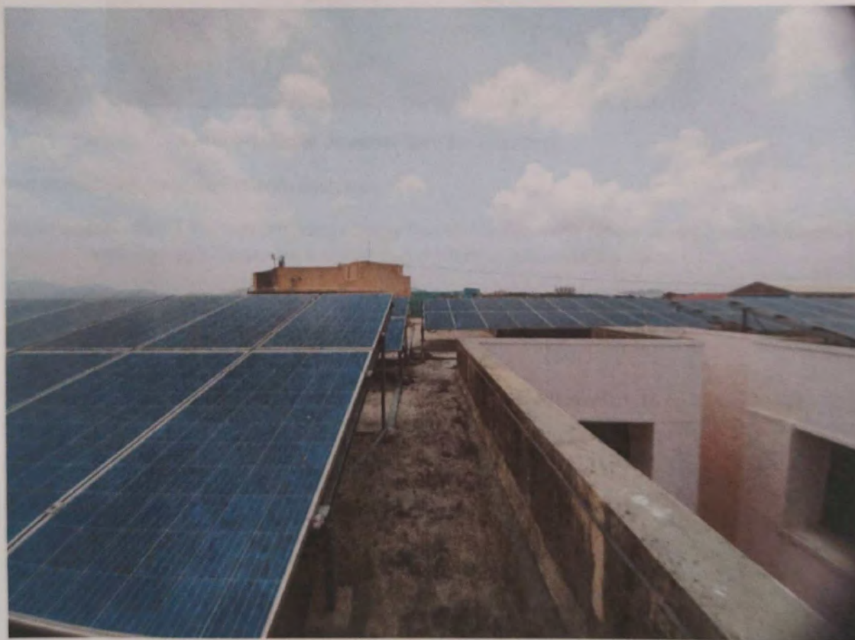
Photo-5: 221 kW solar roof top on Siddhant College of Pharmacy building roof.
