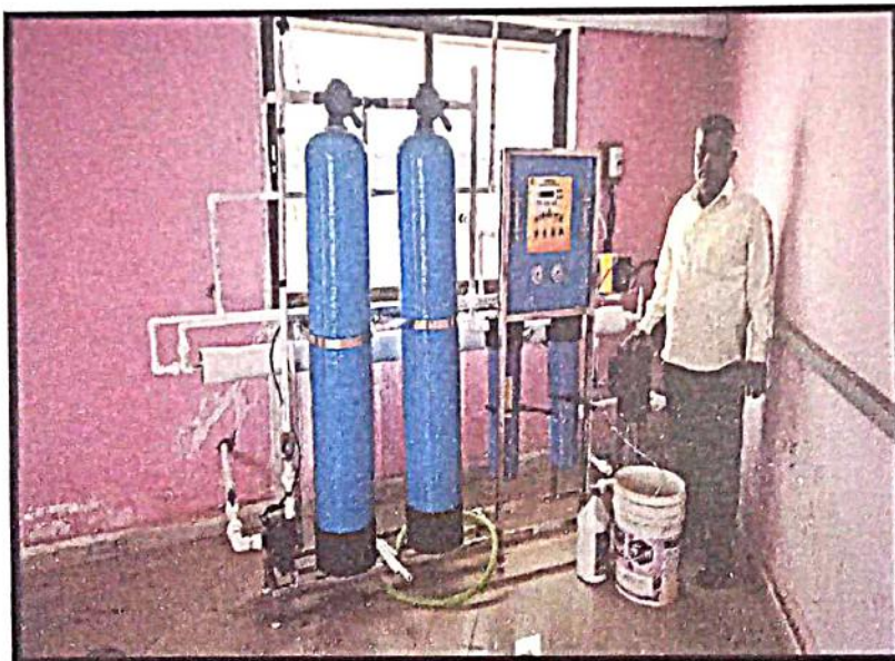
SCOP have RO plant for Purification of water
