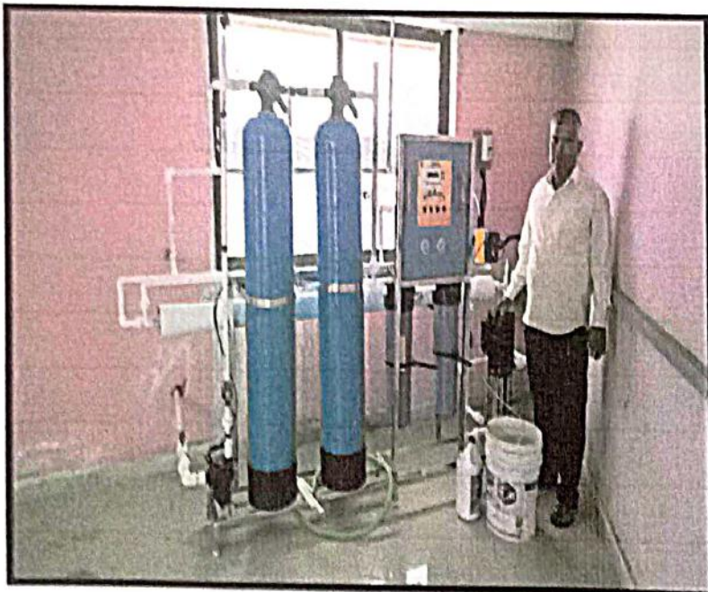
SCOP have RO plant for Purification of water
